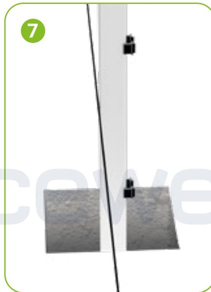
**Place the post in the hole.** Check if it is level and taut against the stretched wire. Then bring it into the ground to the correct height. Use one if necessary post driver. The multi-post generally goes 60 cm into the ground. We recommend keeping the fencing minimal 5 cm above ground level to place.
